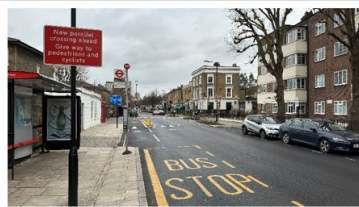
Southgate Road – parallel crossing with segregated with flow cycle lane.
