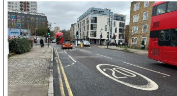
Southgate Road – traffic light controlled junction with cyclist with feeder lane. ASLs encourage cyclists to undertake HGVs in left hand blindspot. Cyclist behaviour may be unpredictable. Pedestrian zebra crossing after junction.
