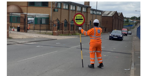
Figure 10 - Correct use of Stop Works signage
