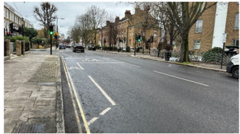
Southgate Road – cyclist ASL feeder lane. ASLs encourage cyclists to undertake HGVs in left hand blindspot. Cyclist behaviour may be unpredictable. Risk of collision is HIGH . Trixi mirror is installed to assist driver vision of vulnerable road users in blind spots.
